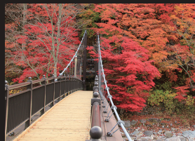
紅吊橋 Kurenai Suspension Bridge
