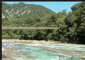
七岩吊橋 Nanatsuiwa Suspension Bridge
