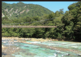
七岩吊橋 Nanatsuiwa Suspension Bridge
